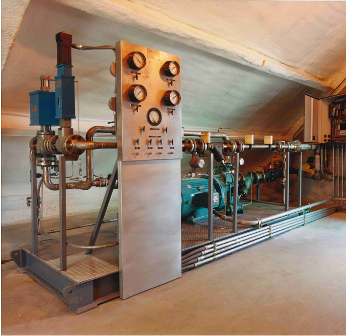
Installation of a water injection pump and flow control skid for a Frame 7 gas turbine gen set in utility service.
